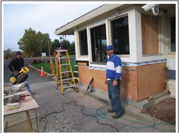
New access window at the South Gate.
