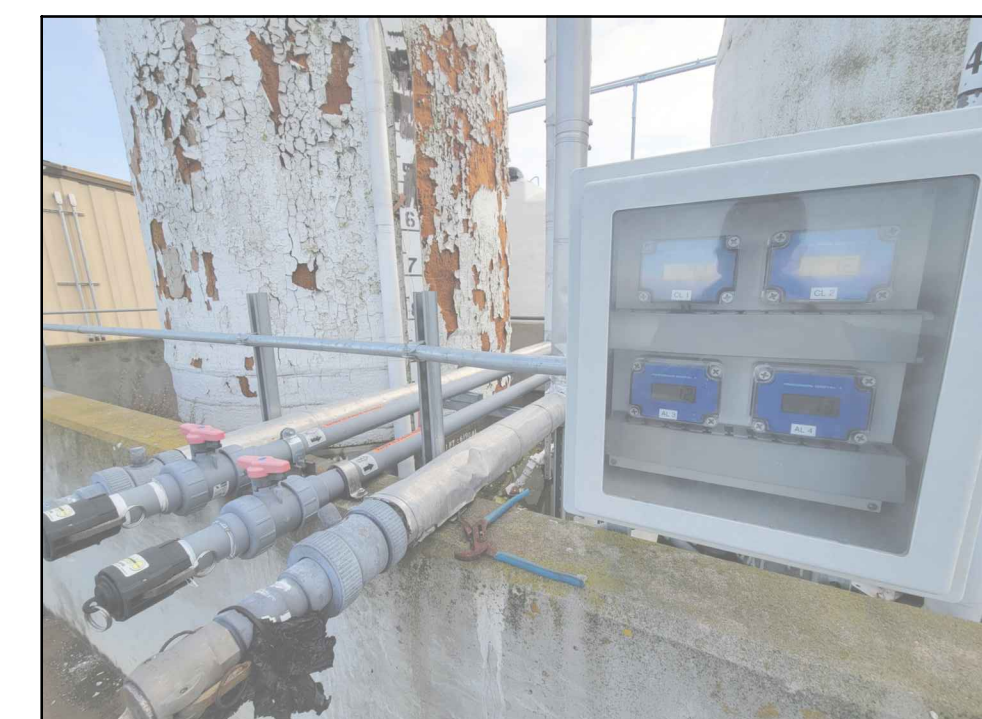
IMAGE NO. 4 CHEMICAL TANK UNLOADING STATION / TANK LIQUID LEVEL PANEL
