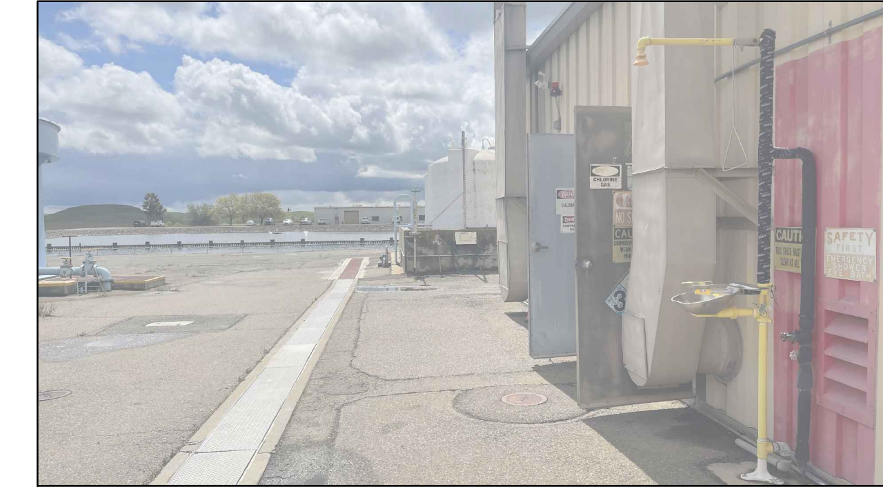
IMAGE NO. 2 CONTROL BUILDING UTILITY TRENCHES
